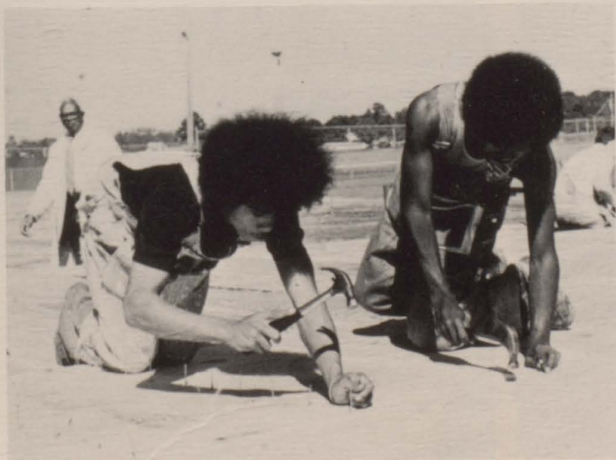
MAKING HIS ROUTINE checks, Mr. Bell observes Darrelle Banks, Kenneth Lee, and William Orr working on the floor.
